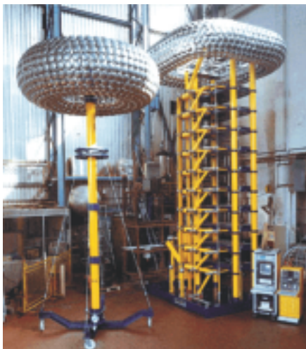
GTN-Impulse Generator; 200kV/stage, 2000 kV-100kJ
